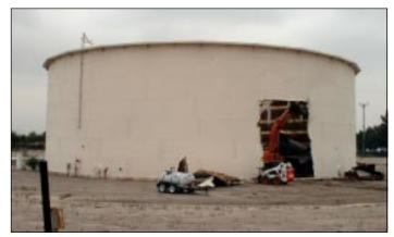
Completed Access Hole. The access holes cut into the tanks are large enough to drive a drill rig through to conduct soil sampling.
